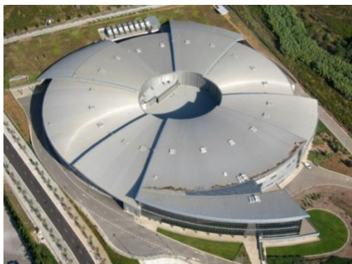
Figure 1. Aerial view of the ALBA Synchrotron Light Source located in Cerdanyola del Vallés (Barcelona, Spain).
